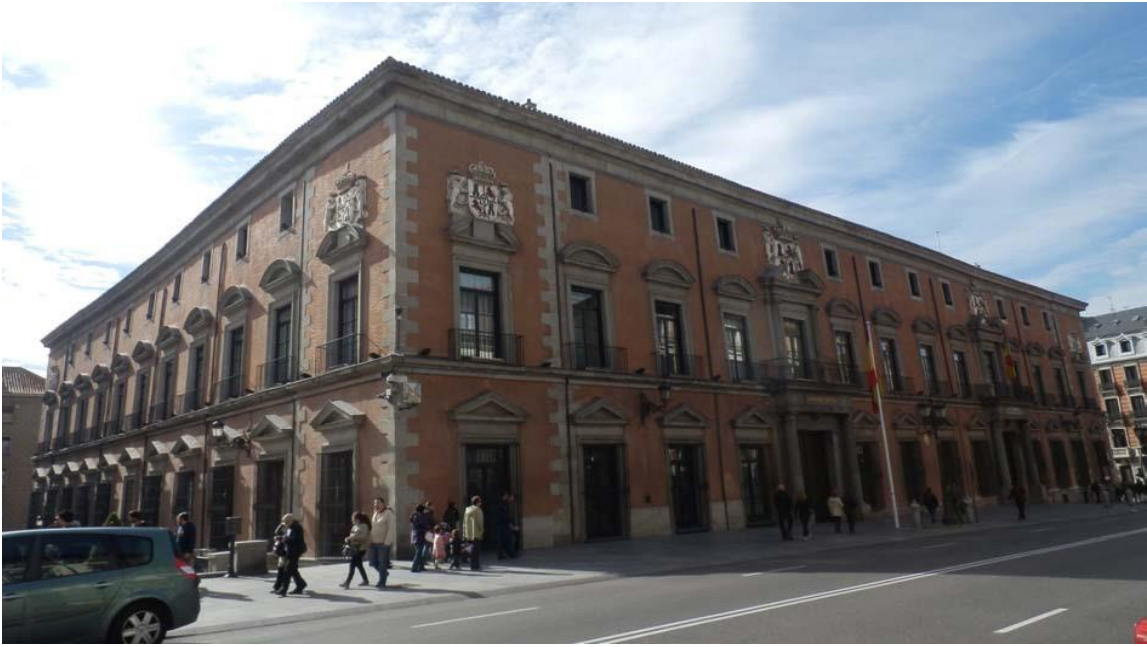
Facade from the Palace of Uceda.
